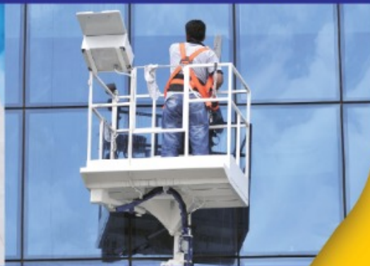
External Glass Cleaning with Cradel
