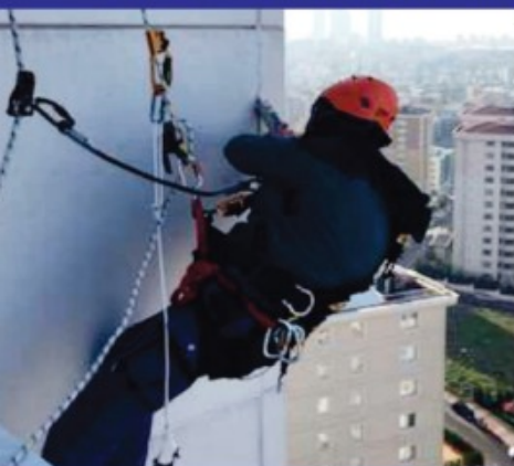
Light Fixing with Rope Access
